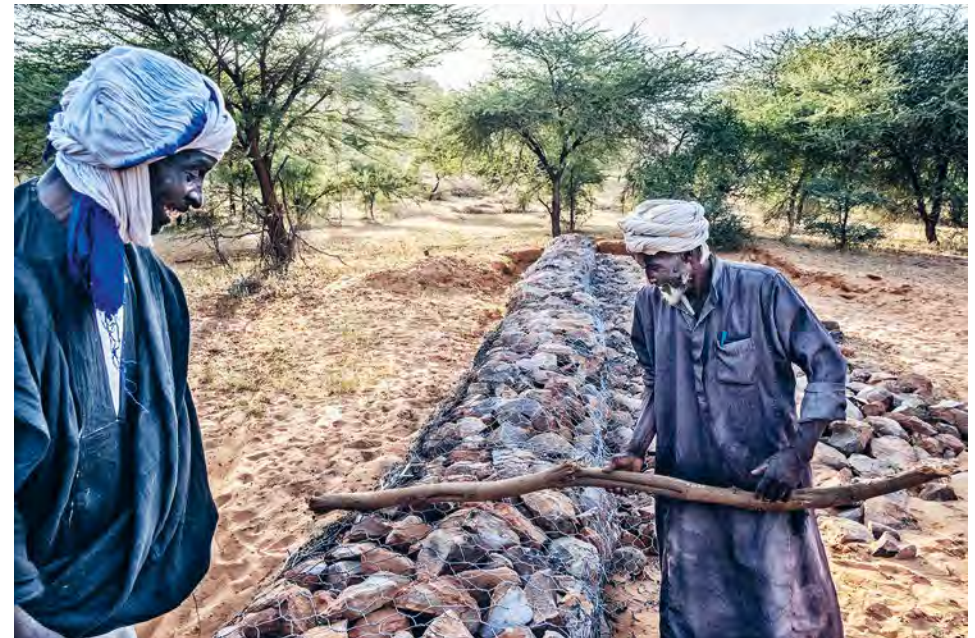
Two members of a local management committee check that the sills used to fight erosion are working properly. Oudey Ejride, Assaba. © Tim Dirven / VSF
